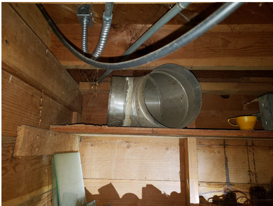
Photo 1. Asbestos-Containing Duct Felt Tape – Basement Electrical Equipment Storage
