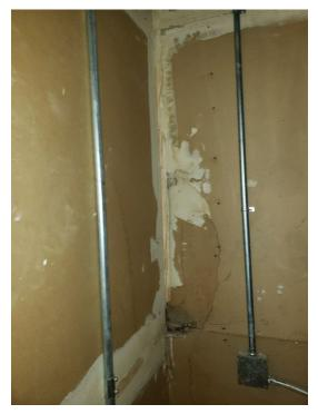
Photo 10. Damaged Gypsum Board/Joint Compound Wall in Upper Gym Mechanical Room
