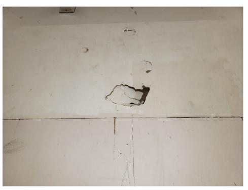
Photo 9. Damaged Gypsum Board/Joint Compound Wall in Upper Gym over Boy's Locker Room
