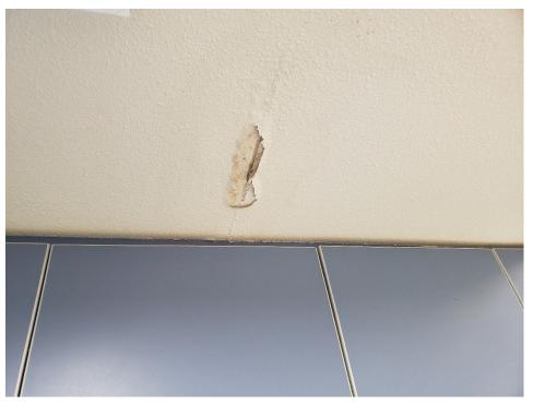
Photo 7. Damaged Gypsum Board/Joint Compound Soffit in Room 3
