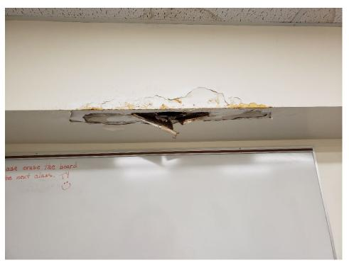
Photo 5. Damaged Gypsum Board/Joint Compound Soffit in Conference Room
