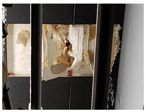
Photo 1. Damaged Gypsum Board/Joint Compound Ceiling Material in Theatre Backstage Area
