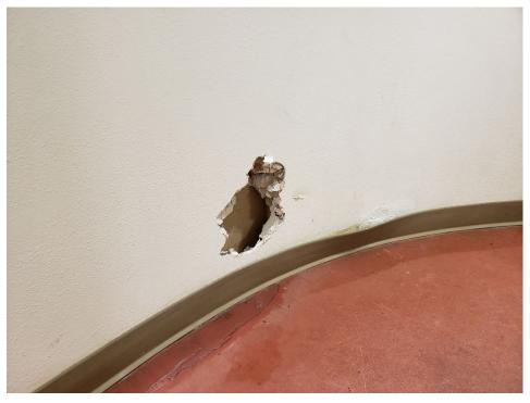
Photo 4. Damaged Gypsum Board/Joint Compound Wall in Women's Restroom
