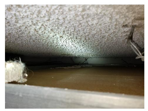
Photo 8. Damaged Spray-on "Popcorn" Ceiling Texture concealed above lower Suspended-grid Ceiling in Room 2
