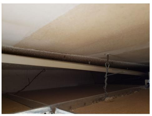
Photo 3. Spray-on "Popcorn" Ceiling Texture concealed above Suspended-grid Lower Ceiling in Room 13
