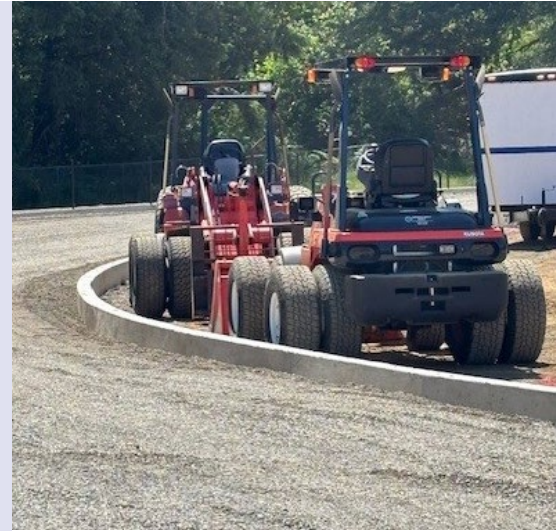
Inner and outer curbs set for track
