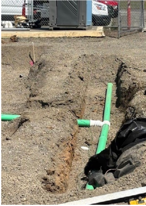
Extensive storm drainage required for field, plaza, and out buildings.
