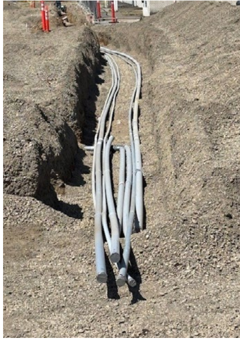
Line power and low voltage conduits ran under paved plaza for lighting, sound, timer, and out buildings.
