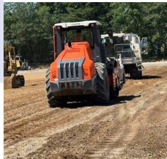
Grounds required cement-treatment
